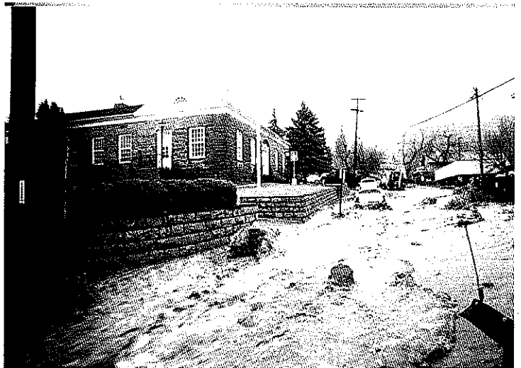
Manitou Springs - 1999 Flood
