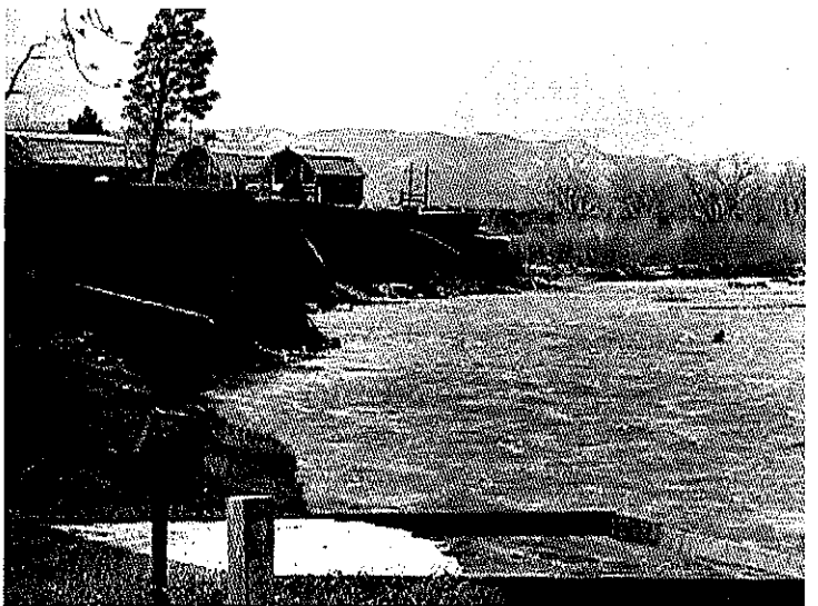
Bank erosion on Fountain Creek
