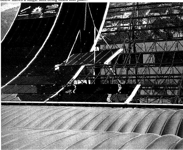
This reduces installation costs, and when coupled with greater insulation thickness as found in S.O.L.I.D. collectors these large collectors are also able to achieve temperatures in excess of 230F.
