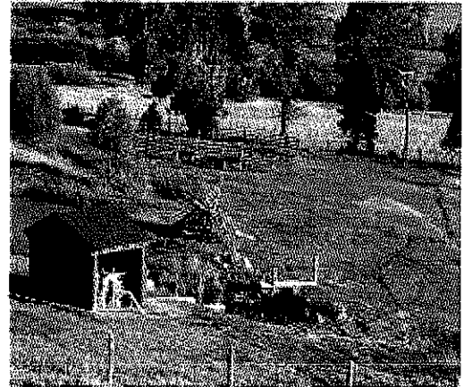
ACRE's Micro-Hydro Project at Elk View Ranch in Archuleta County Completed November 2008
