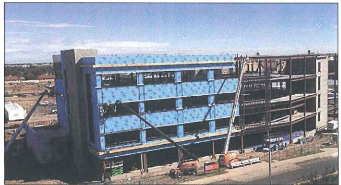
Bioscience II In Construction
