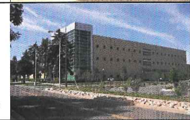
Campus Services Building
