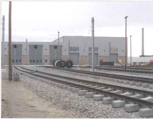
Large bifold doorways allow commuter rail vehicles to enter the maintenance building with overhead power.
