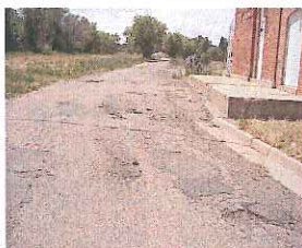
Existing Roadway Condition
