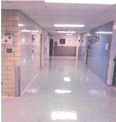
Typical wall condition, Meyer Building
