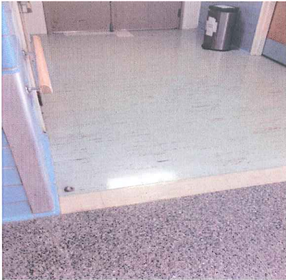
Typical floor condition, Meyer Building
