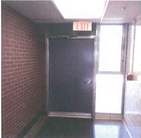
Typical door conditions, Meyer Building
