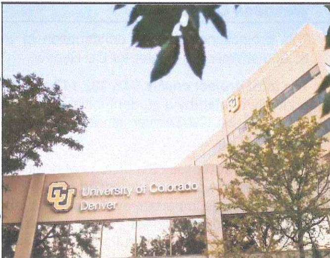
Image of CU Denver Building
