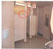
Colorado Mental Health Institute at Pueblo, Bldg. 116 Shower Room - Pre-Mitigation
