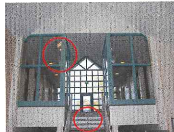
Lookout Mountain Youth Services Center Glass Wall - After Mitigation
