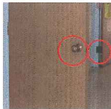
Colorado Mental Health Institute at Ft. Logan, F-Cottage Door Hardware - Pre-Mitigation
