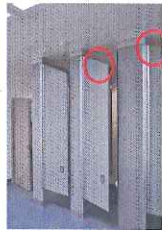
Colorado Mental Health Institute at Pueblo, Bldg. 116 Shower Room - After Mitigation
