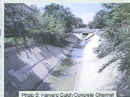
Photo 5: Harvard Gulch Concrete Channel
