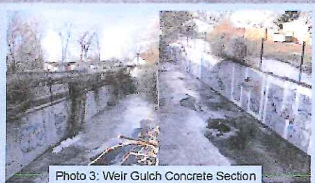
Photo 3: Weir Gulch Concrete Section
