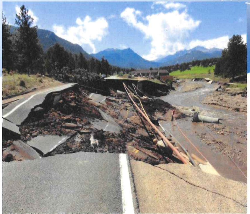
Flood damage near Estes Park, Colorado from the Upper Thompson River.
