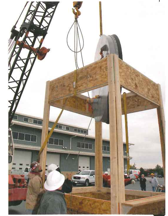
Crews practice bulkhead placement before dive team work begins
