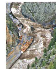
FRONT COVER Dille Tunnel diversion structure in Big Thompson River flood waters; photo courtesy City of Loveland
