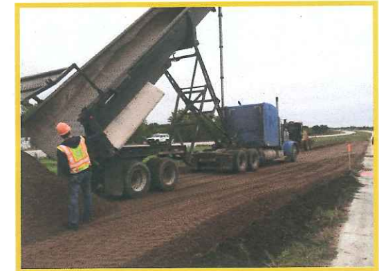
U.S. Highway 34 near Kersey
