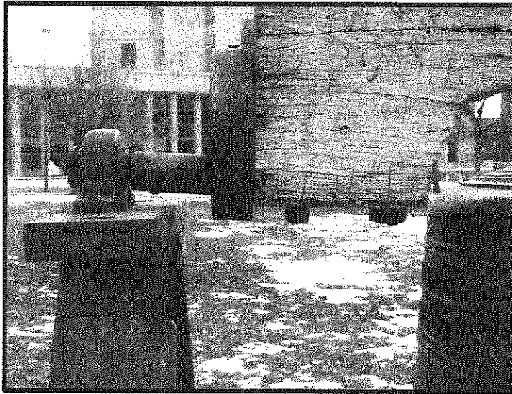
Figure 5. Connection failure at bearing. Both axles have shifted out of alignment resulting in the sagging of the support structure.
