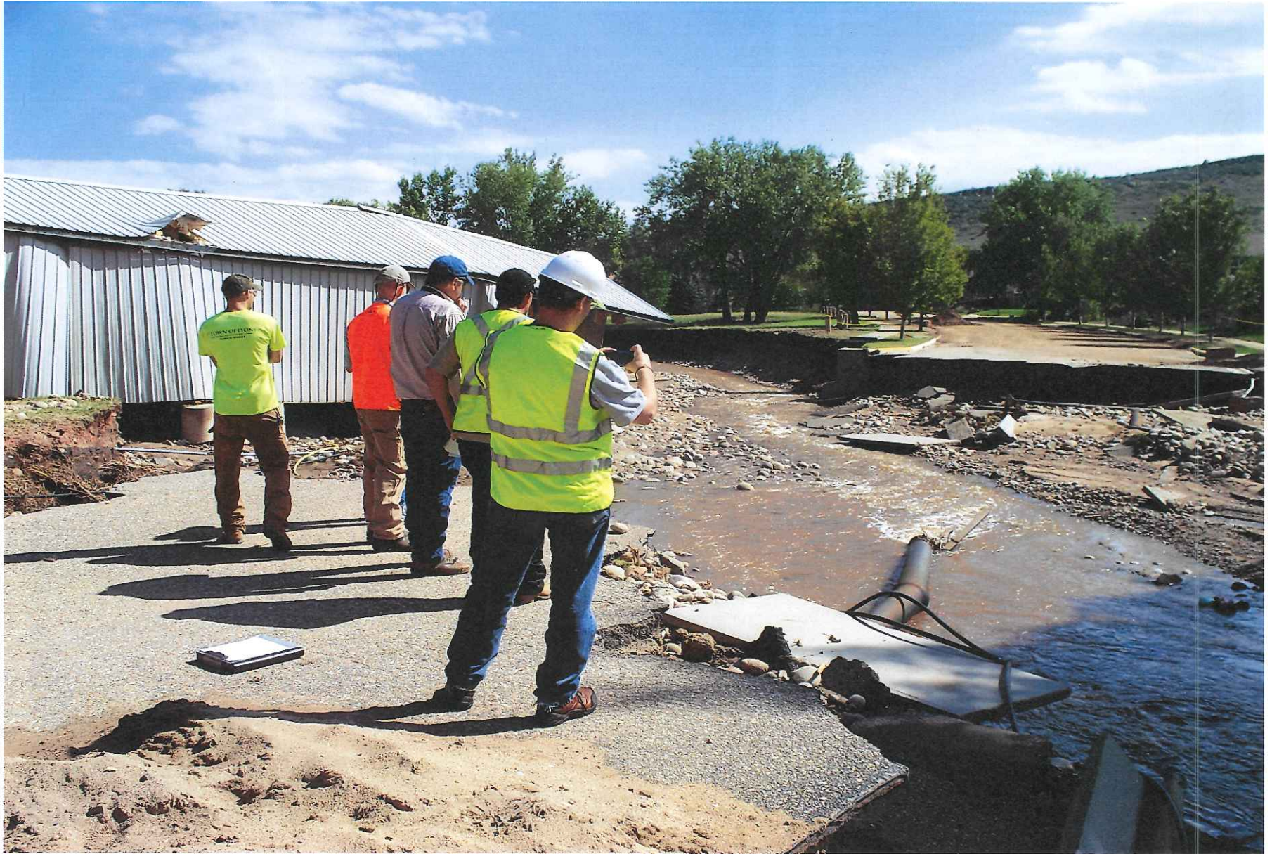
Lyons – WWTP & Exposed Drinking Water Line
