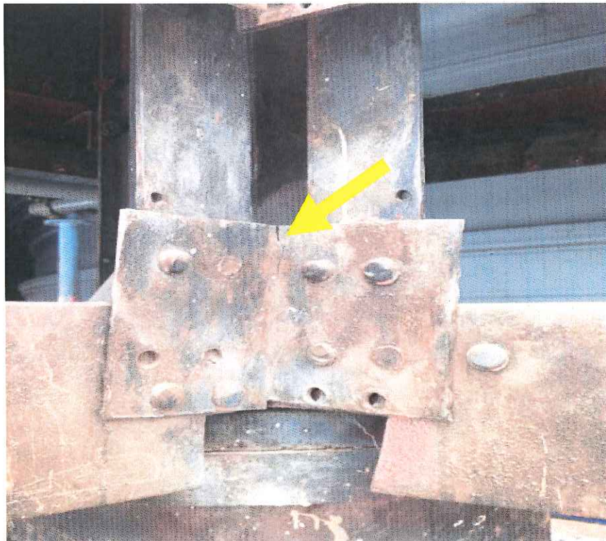
Photo 07.7: Cracked angle
