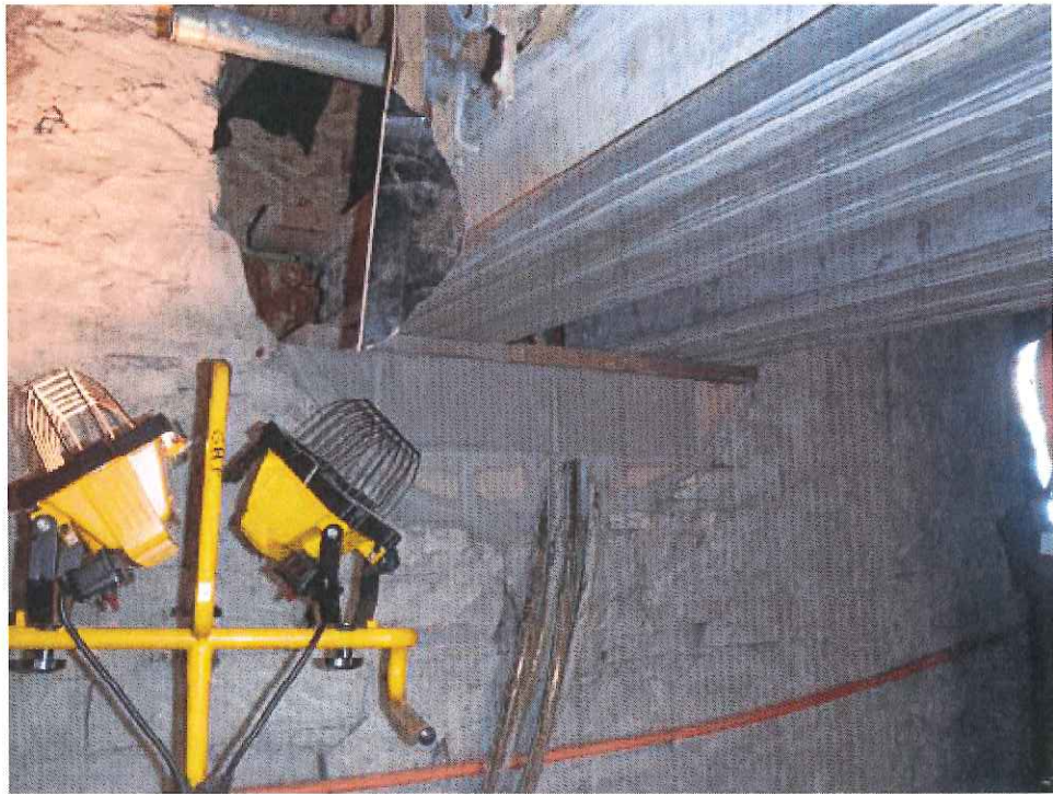
Photo 1.2: Installed radial scaffolding support beams.
