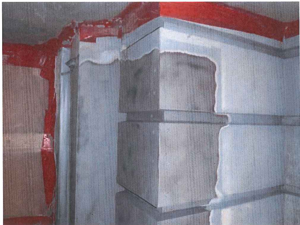
Photo 1.3b: Coatings removal mock-up.
