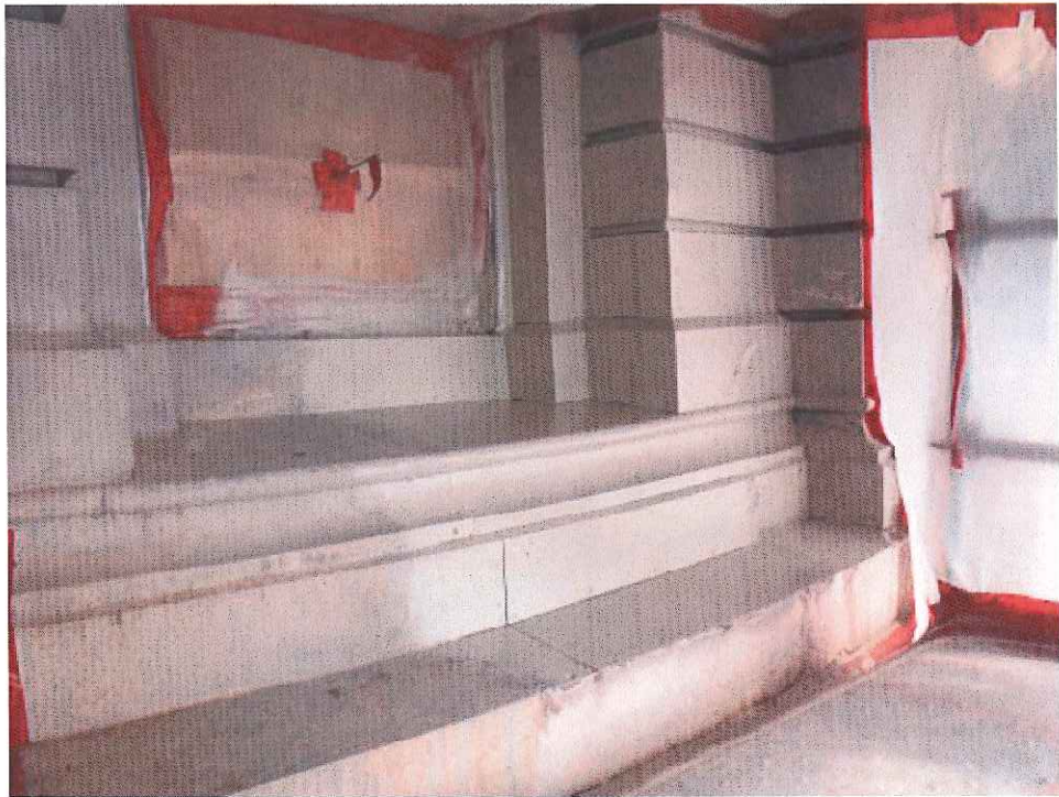
Photo 1.4: Prime coat mock-up.
