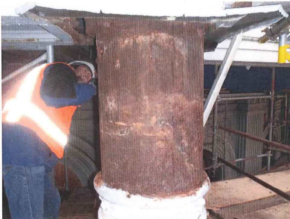
Photo 1.7a: Removed column capital.
