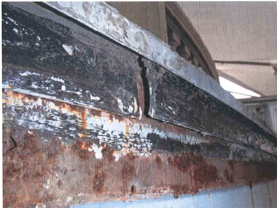
Photo 1.6b: Fibrous strip backing behind gutter.
