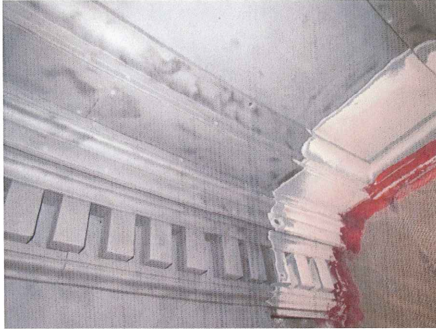
Photo 07.6: Cleaning of soffit below upper terrace
