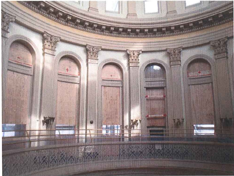
Photo 1.9: Installed window protection – observation deck.
