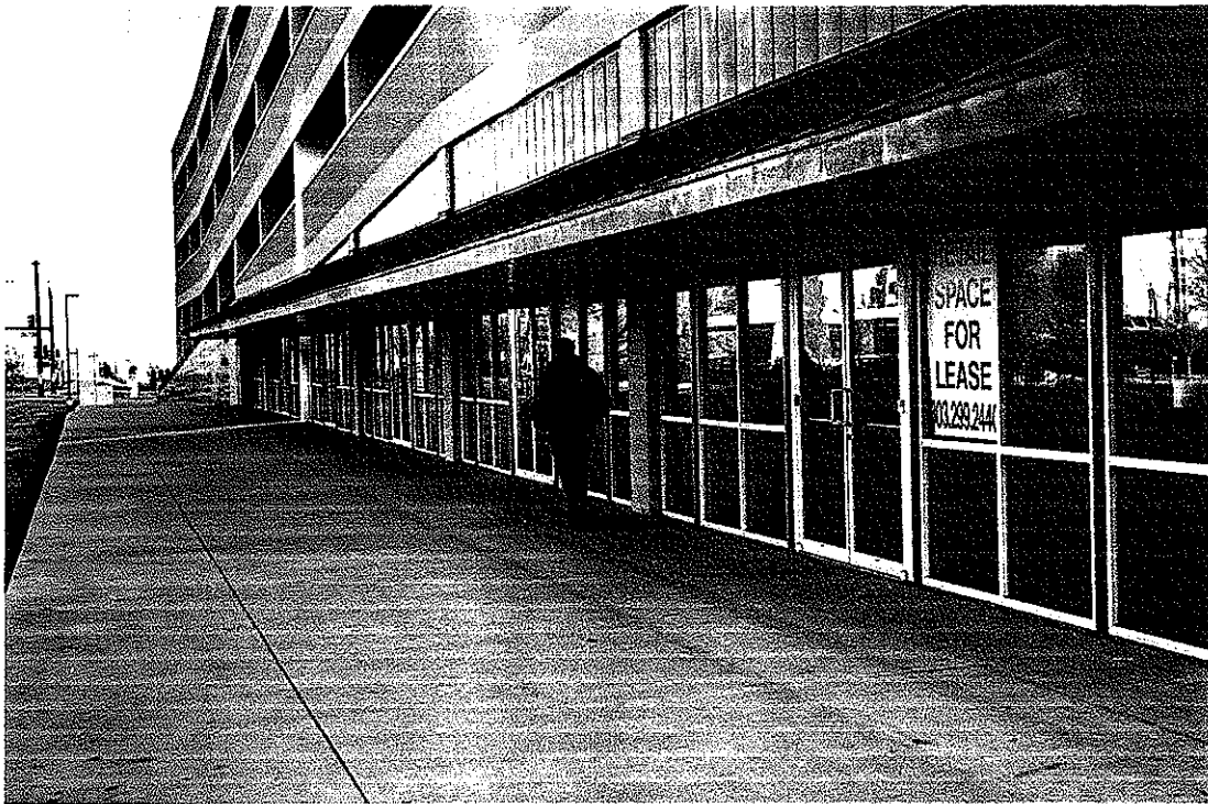
RTD PARKING GARAGE 2 GROUND FLOOR - EMPTY FOR 5 YEARS
