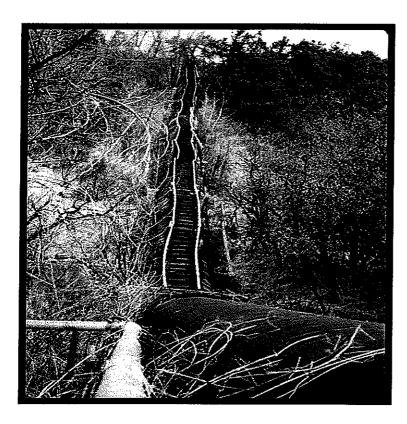
Last replaced in 1938, this siphon on the Grass Valley Canal was losing water and in danger of failing.
