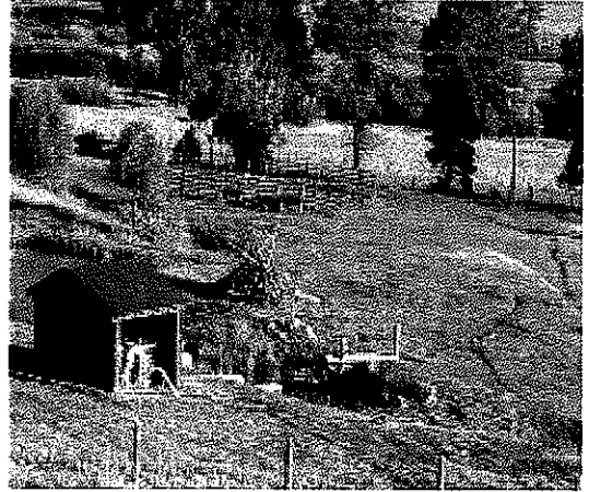
ACRE's Micro-Hydro Project at Elk View Ranch in Archuleta County Completed November 2008
