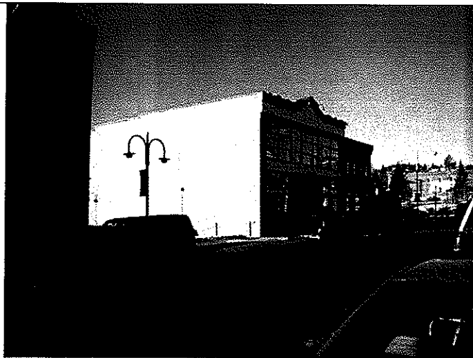
Aspen Mine -- $3-5 million abandoned casino building now used for delivery of social services
